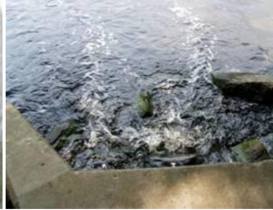
Final Effluent at Wisconsin River
